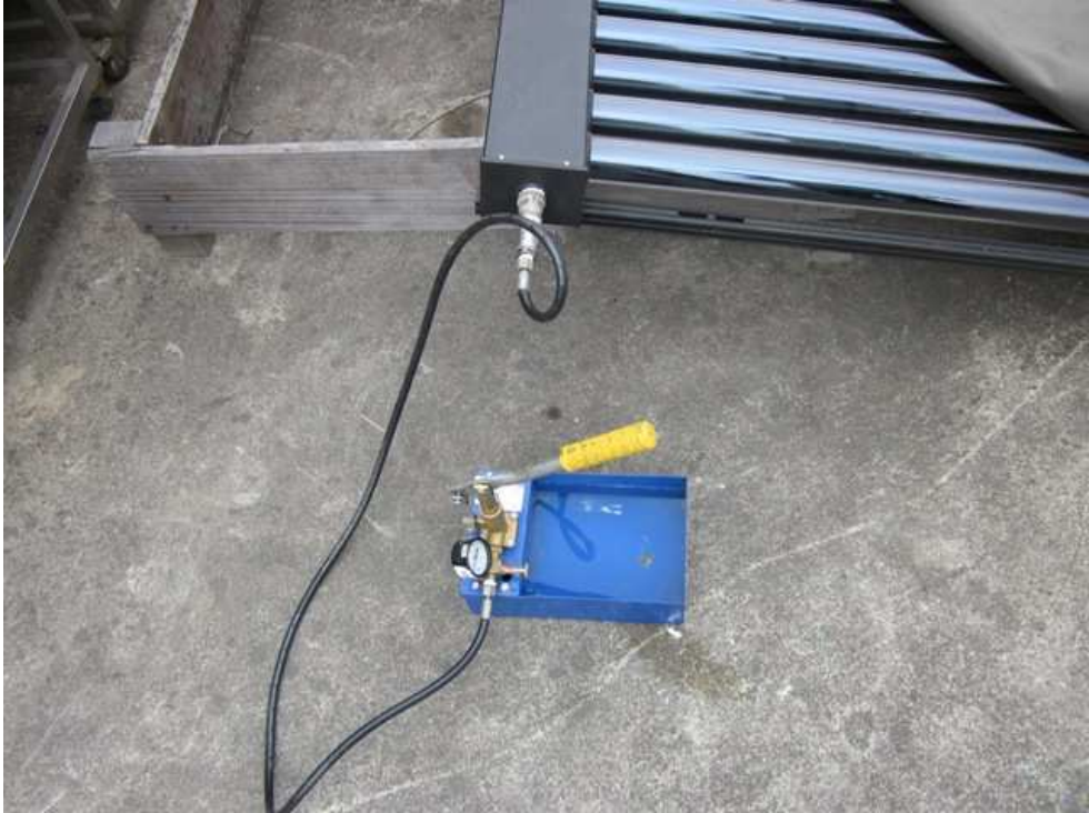
Figure- C.1: Photo of internal pressure test
